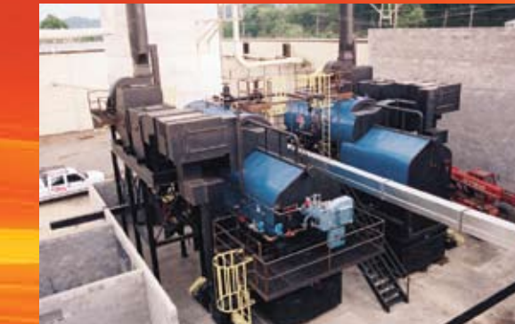
Twin 600 BHP Hardwood veneer plant Steam vats and "coil" dryer heat application.
