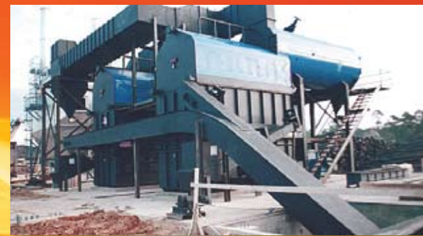
Twin 1200 BHP Saw Mill / Arkansas
