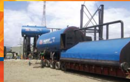
Twin 1200 BHP "Super Heated" 450psi Erected in Dominican Republic.
