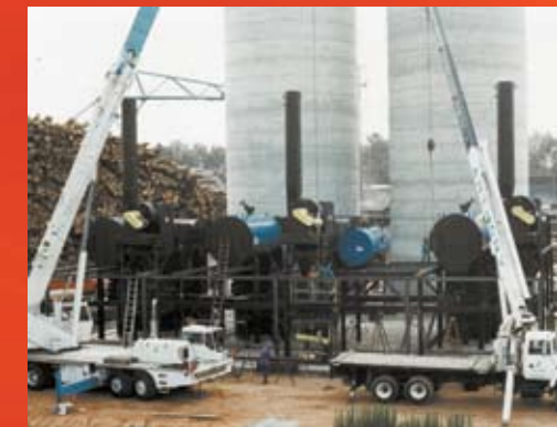
Triple 600 BHP "Pine" Saw Mill Steam "coil" dry kilns heat application.
