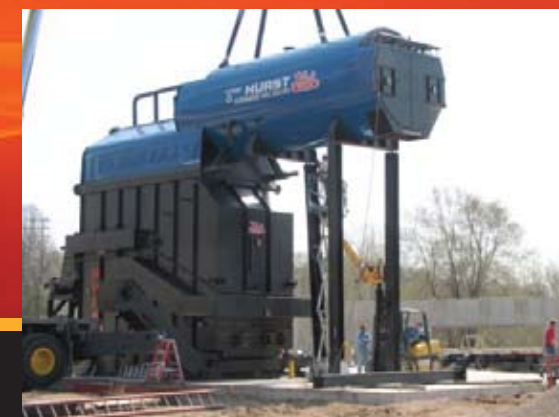
1500 BHP 1500 BHP 250 psi design being erected in Wisconsin. This assembly is shipped in (3) large modular pieces for a cost saving installation.
