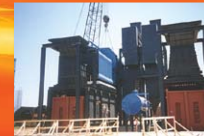
1500 BHP 1500 BHP 250 psi design being erected in Wisconsin. This assembly is shipped in (3) large modular pieces for a cost saving installation.
