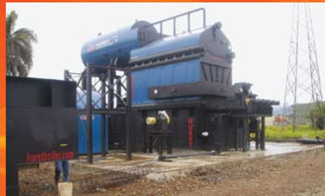
1200 BHP (Traveling Grate Stoker)
